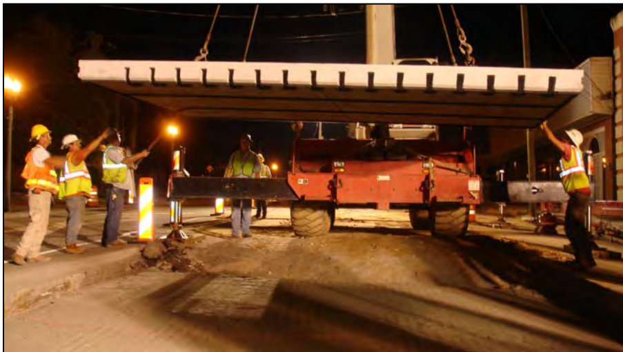
Placing First Slab
