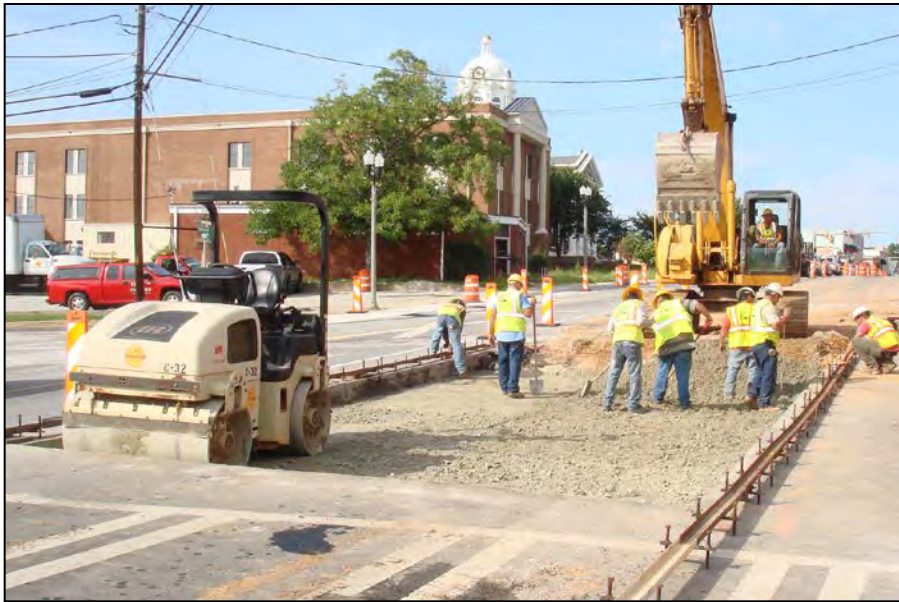
Grading and Compacting New Aggregate Subbase
