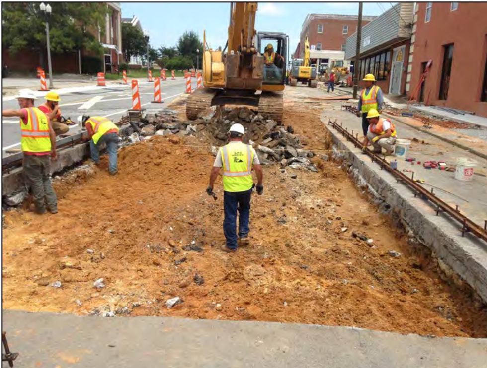
Removing Multiple Layers of Old Pavement
