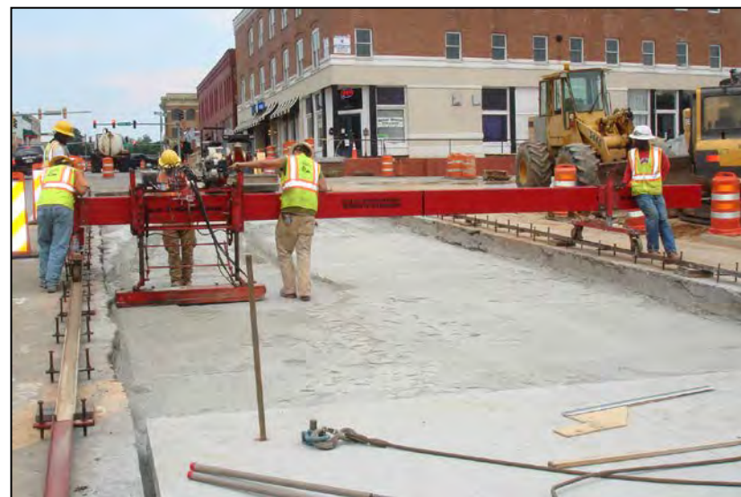
Super-Grading With Hand Operated Grader (H.O.G.) to +/- 1/8" Accuracy
