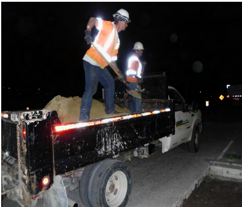
Laborers Shovel Stone Dust into Patch
