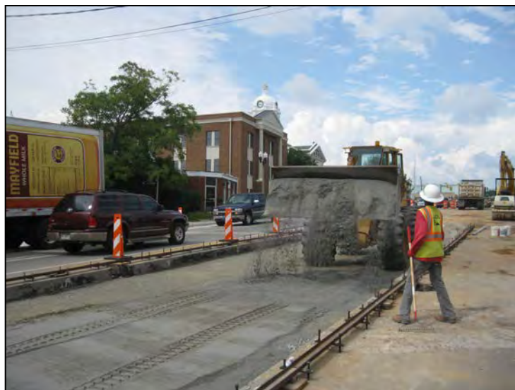
Installing Bedding Material Over Aggregate Base
