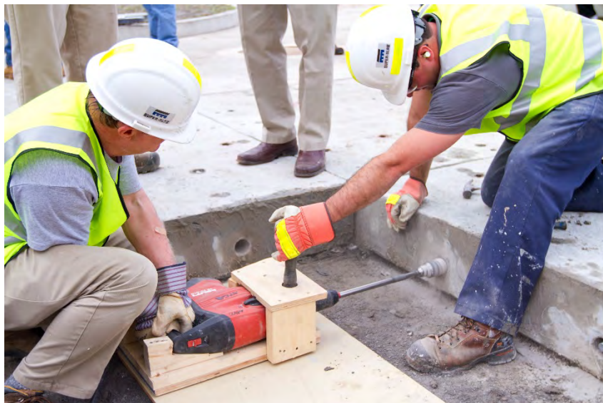
Core and Remove Coupler
