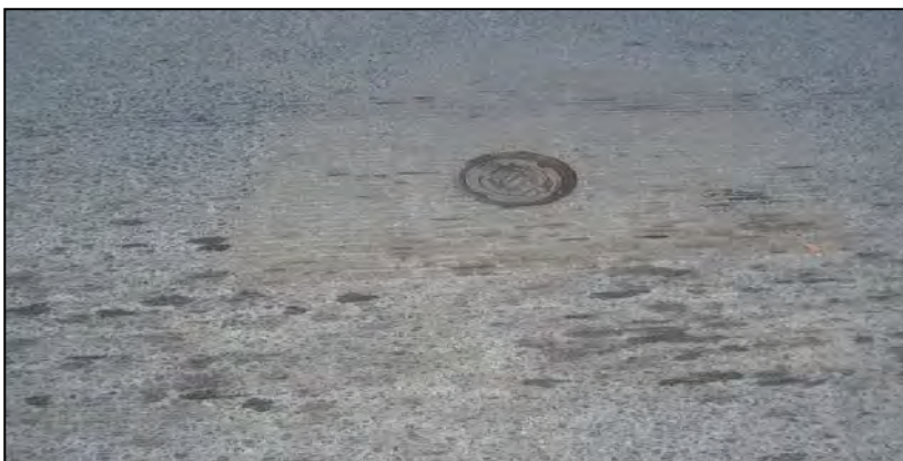
Water Valve – CIP Closure Pour
