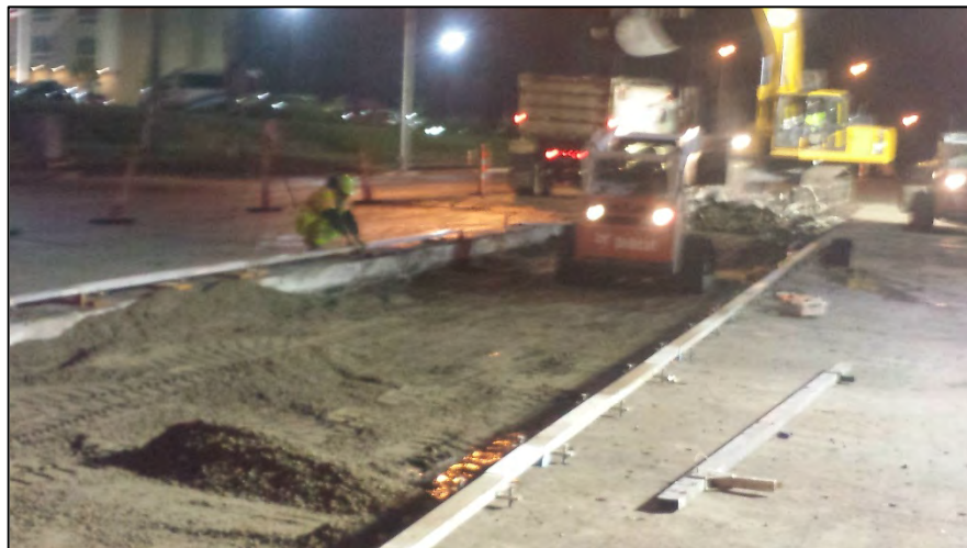
Removing Old Base, Placing New Cement-Treated Bedding Material
