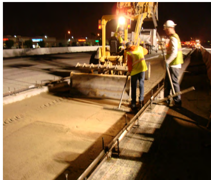
Stone Dust can be placed with heavy equipment
