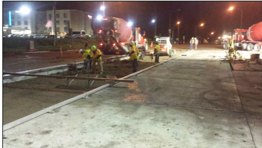
Grading Cement-Treated Bedding Material
