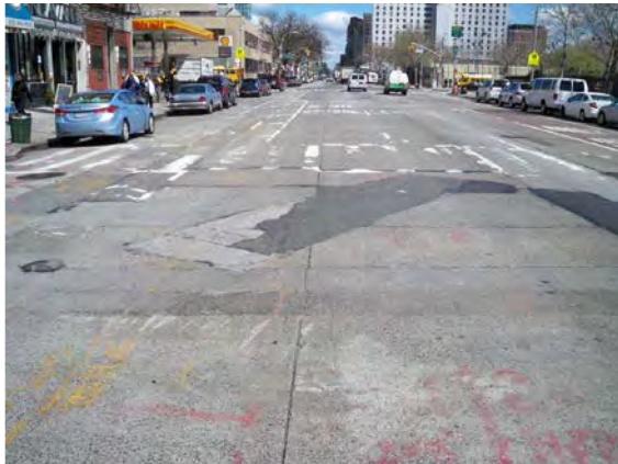
Randomly Cut, Remove and Replace Pavement
