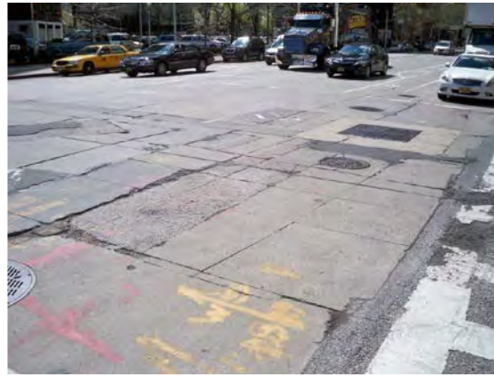
Randomly Cut, Remove and Replace Pavement
