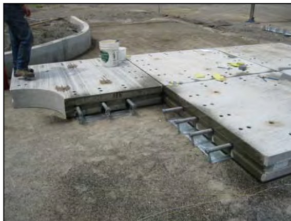
Independent Dowels Placed in Slots
