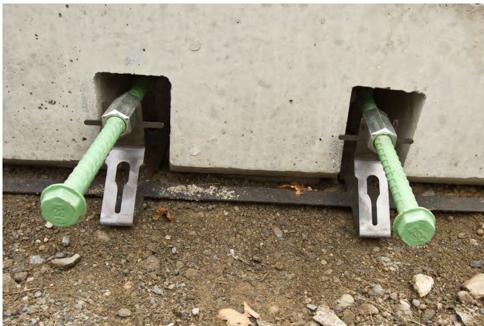
Removable/Replaceable Longitudinal Joint Tie
