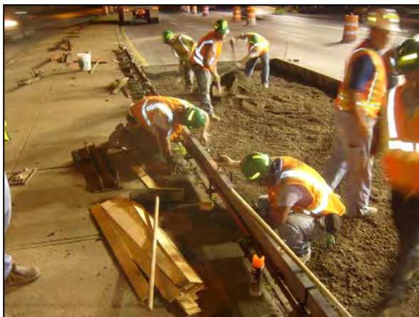
Setting Grading Rails
